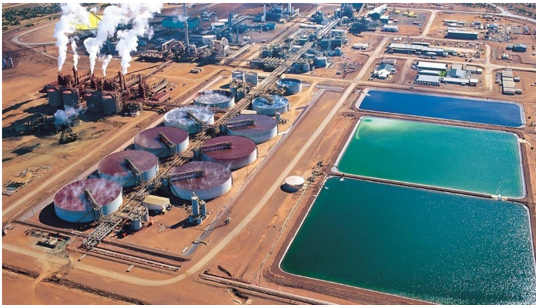
Figure 2: Glencore's Murrin Murrin hydrometallurgical plant in Australia.
